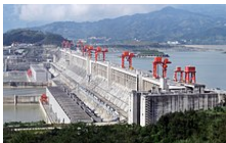
The Three Gorges Dam on the Yangtze River in China
